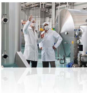
Pharmaceutical water treatment
